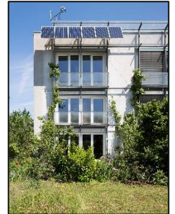
The world's first Passive House building in Darmstadt, Germany. © Peter Cook
