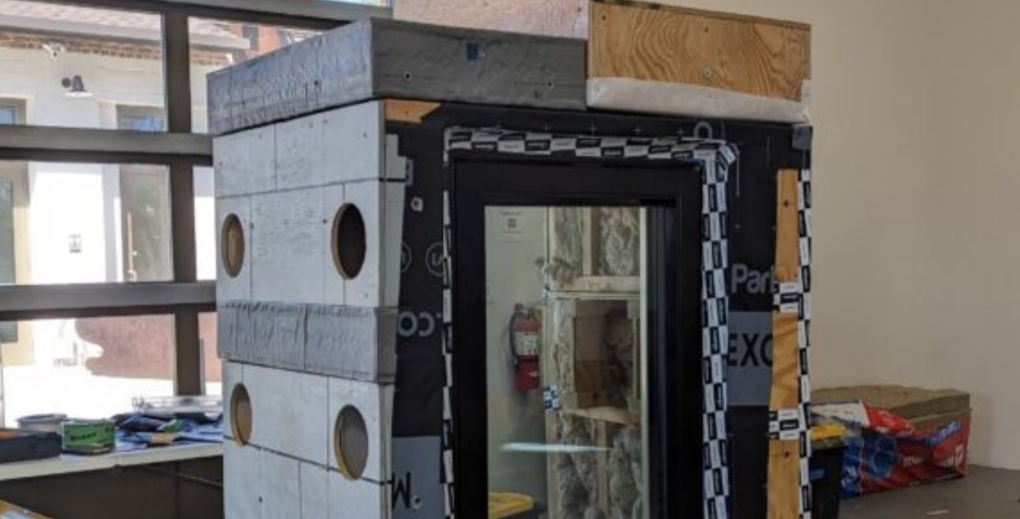
Passive House Pod Built by Kelly Hsu and Team in Santa Barbara
